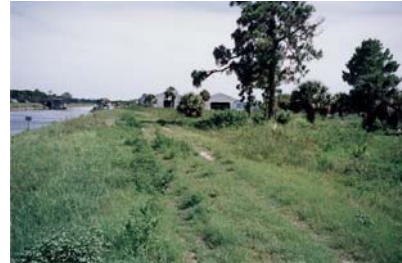
ICWW to the East (view to the south)
