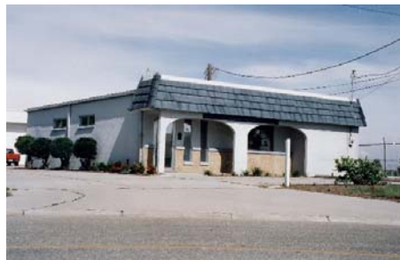
WCIND headquarters with paved parking lot
