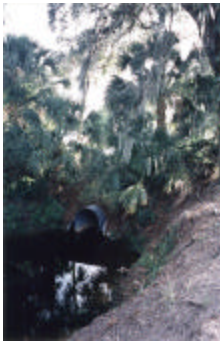
Site S-WCIND-P2 - 4 ft Culvert passing under Cortina Drive.
