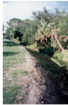
Stormwater drainage ditch. (looking northeast toward Baveno Drive towards north end of easement)
